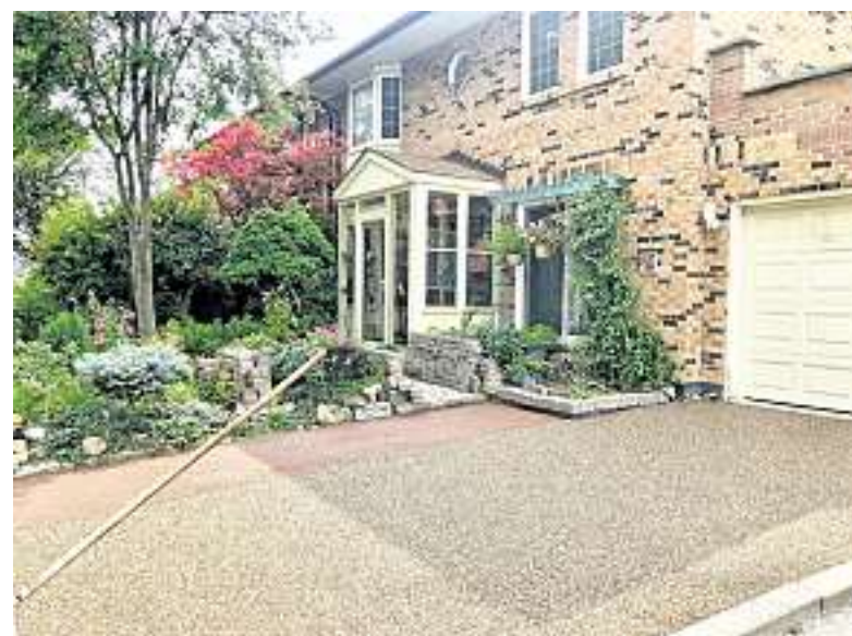
Scarborough homeowners shared a new pathway project between their houses to clean it up and eliminate water issues with an anti-slip surface.
